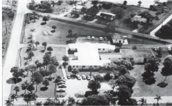
This aerial photo shows Charlotte Community Hospital in Punta Gorda (later, Charlotte Regional Medical Center, then Bayfront Health, now ShorePoint Health) prior to its expansion in 1965. COURTESY PHOTO
